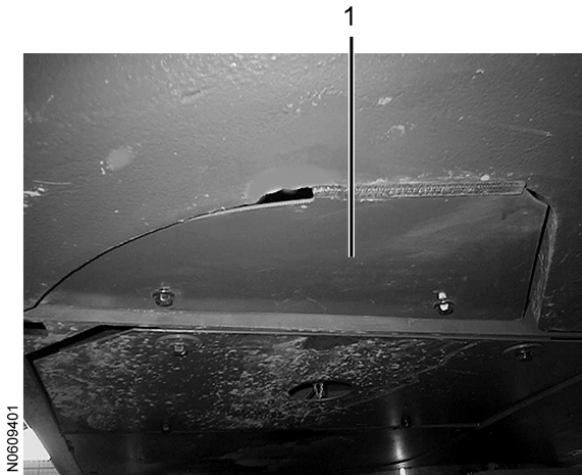
Figure 5 Inspection cover, underside of counterweight
