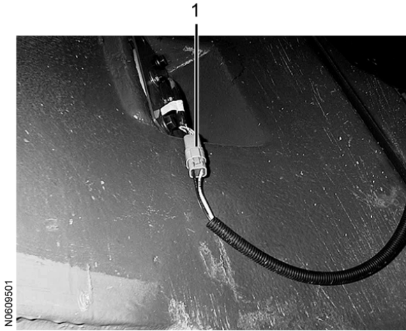
Figure 4 Inside of counterweight
